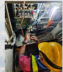
Electrical Panel Upgrade
