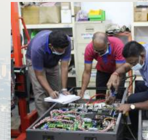
AC/DC Drive Repair
